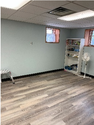
Bell Choir Room - New laminate flooring and vinyl baseboards were installed.
